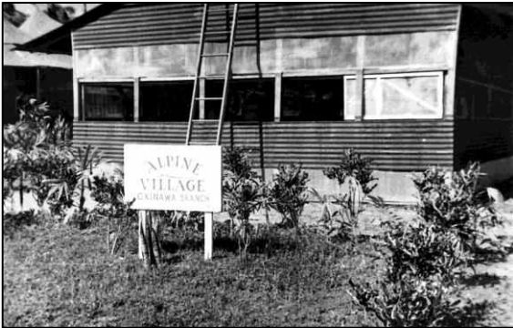
Alpine Village, Okinawa mess hall. Ladder was property of electricians, not permanent fixture.
