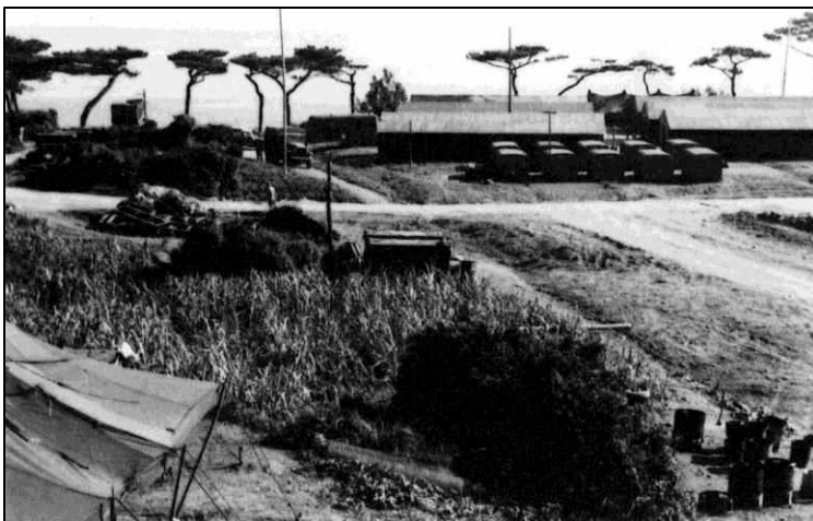
Operations Building and TC-8s, TC-9s.
