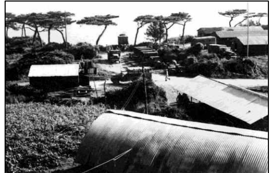
Power Generators, Carpenter Shop, and Barber Shop (in the foreground).
